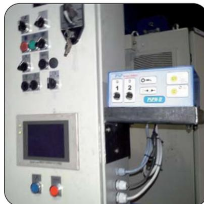
PSP 30 installed out of control cabinet
